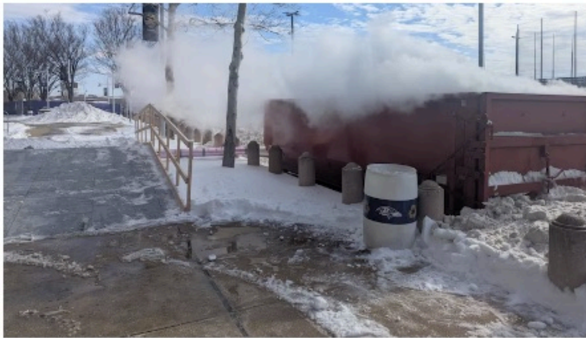
Steam lines hooked up to a dumpster helped the Maryland Stadium Authority melt snow following the Jan. 25 snowstorm. (Maryland Stadium Authority Facilities)
